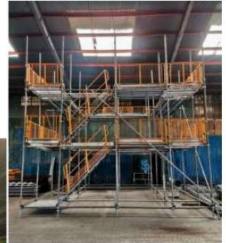
PIPE ACCESS SCAFFOLD
